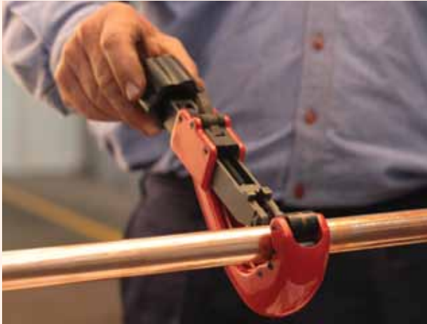
1. Cut copper tube to length using a pipe cutter.
