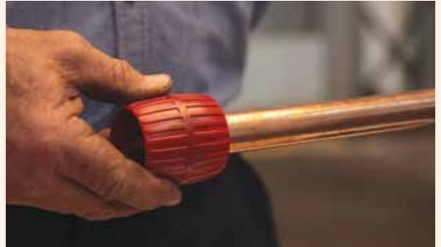
2. Deburr carefully the end of the tube on the inside to minimize turbulence and pressure loss according to AS3500 and on the outside to avoid damaging the O-ring.
