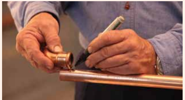
4. Mark the insertion depth by lining up the fitting side by side with the tube and mark the tube. When the fitting is inserted onto the tube the outer edge of the fitting must line up with the marking. For correct insertion depths see column e , table 1, page 17.
